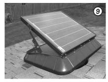
10.) Replace the 7/16" nuts and bolts to lock solar panel in position.
