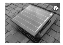
8.) Remove the 7/16" nut & bolt from each support bracket to allow panel to be tilted to desired position.
