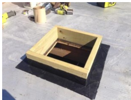
4) Flash curb with membrane.
