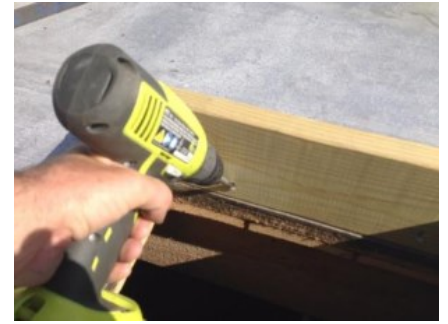
3) Fasten curb to roof.
