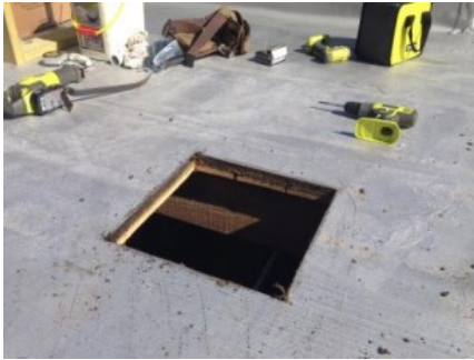
1) Cut 16 1/2" hole through roof.
