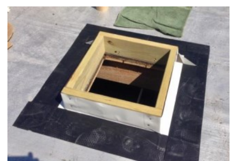
6) Install membrane over metal.
