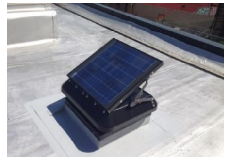
9) Coat flashing with roof paint.
